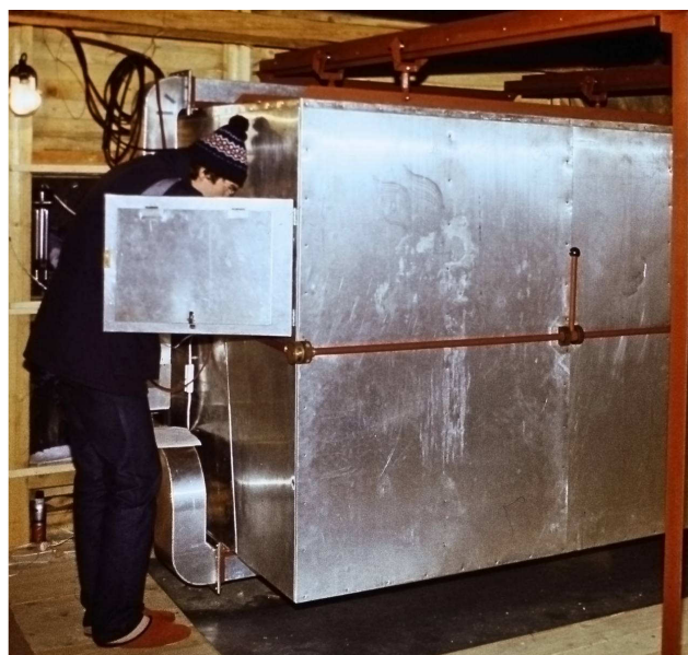
Service of instruments through a door in the container.
