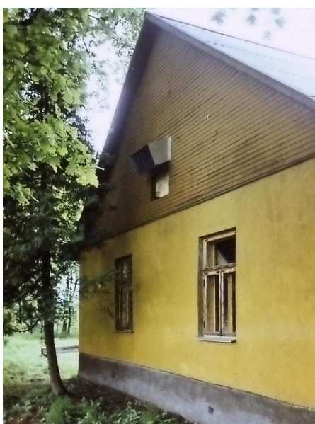
Air intake in the Sepa farmhouse
